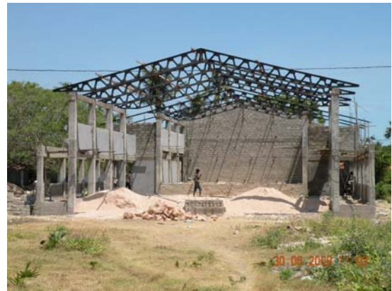
Auditorium under construction June 2009
